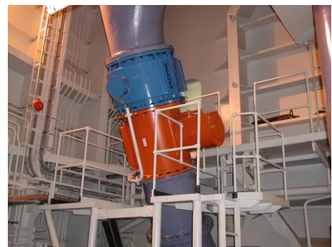
Figure 2: typical application of (orange-coloured) density measurement
